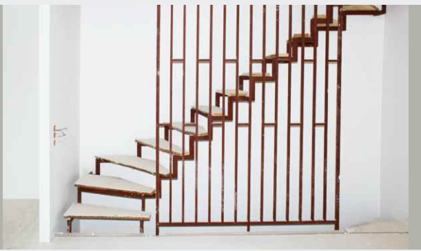
Decoupled harp staircase as skeleton structure
